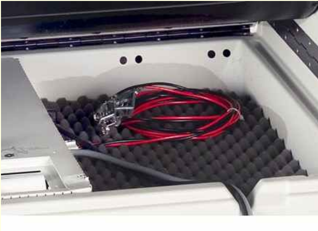
Auxiliary battery connectors
